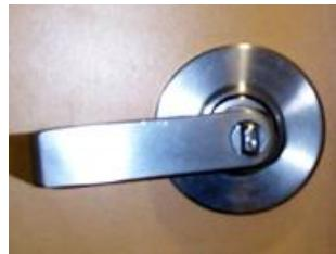
**TYPE 3. Square slot hidden behind metal cap.** Remove cap with fingers. Then use square override key provided by PO&M (image below). Put key in slot and turn.
