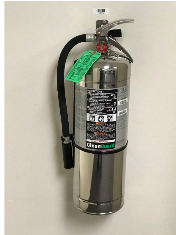
Silver tank is MRI Conditional. Can be brought into the scanner room
