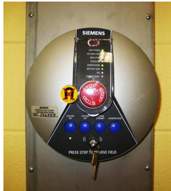
3T Control room Quench button
