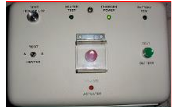
1.5T Scanner room Quench button
