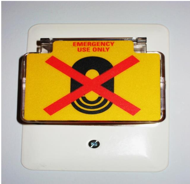
3T Scanner room Quench button
