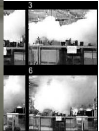
MRI Scanner Superconducting Magnet Quench
