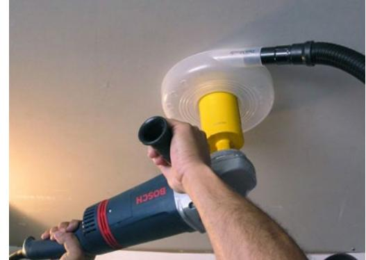
Projects commonly completed using these systems include drilling small penetrations, cutting in for wire receptacles, and placing backing plates for hanging objects from the wall. Because the containment cannot be posted, display the required postings (including the ICRA permit) in the work area.
