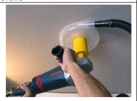
Projects commonly completed using these systems include drilling small penetrations, cutting in for wire receptacles, and placing backing plates for hanging objects from the wall. Because the containment cannot be posted, display the required postings (including the ICRA permit) in the work area.
