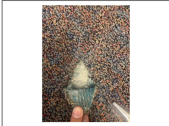
View of the Concrete Foundation Underneath the Multicolor Carpet
