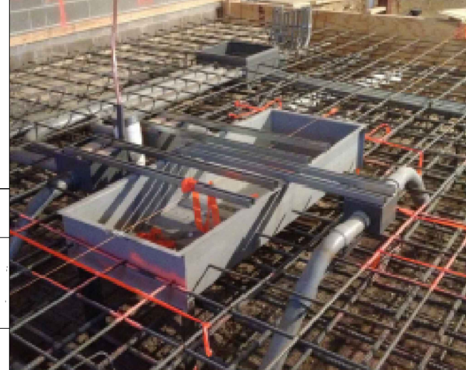
A5 SUB-BASE BEFORE POURING CONCRETE NOT TO SCALE
