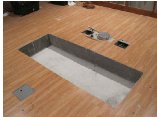
D3 SUB-BASE AFTER POURING CONCRETE NOT TO SCALE
