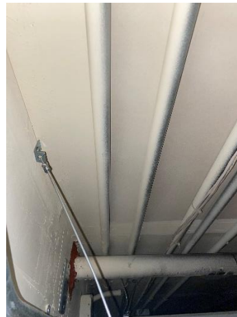
Additional view above ceiling
