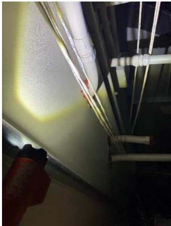
Additional view above ceiling
