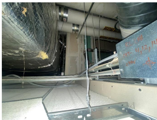
Additional view above ceiling showing fiberglass insulated piping and HVAC ducting
