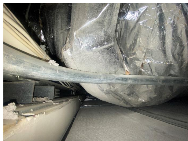
Additional view above ceiling showing fiberglass insulated piping and HVAC ducting
