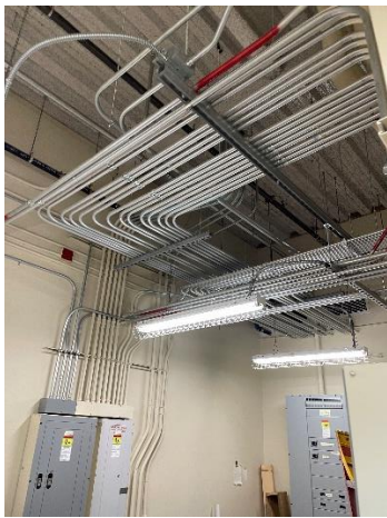
View of the ceiling within one of the telecom rooms
