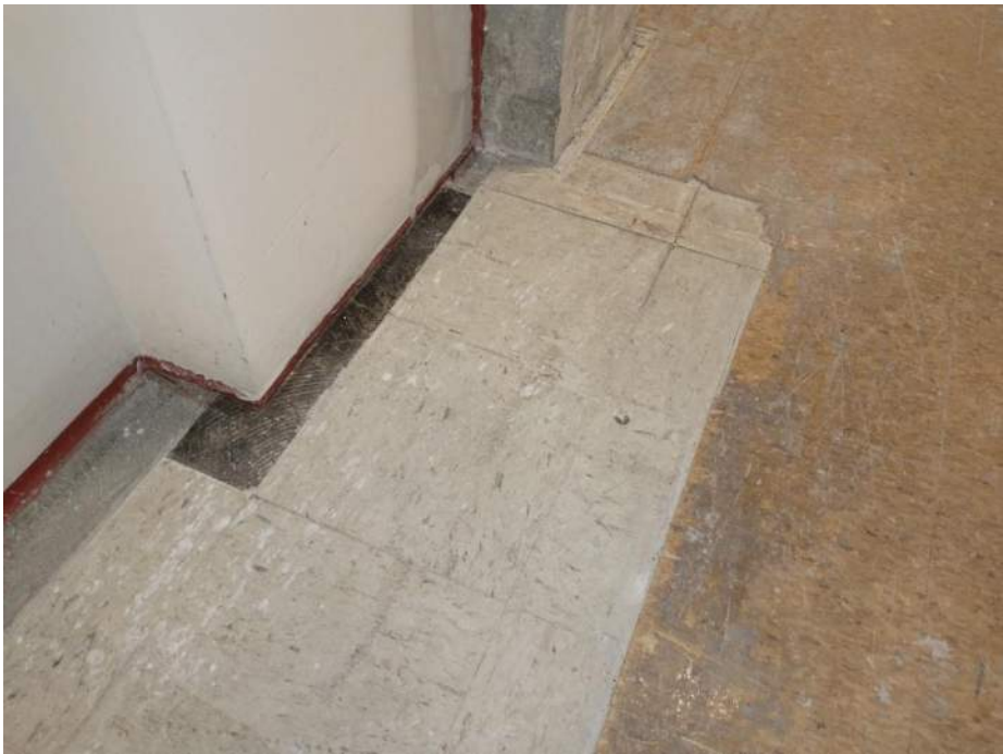
1 st Floor Vacant Space 1119 with visible 9” vinyl floor tile beneath top layer of 12” vinyl floor tile
