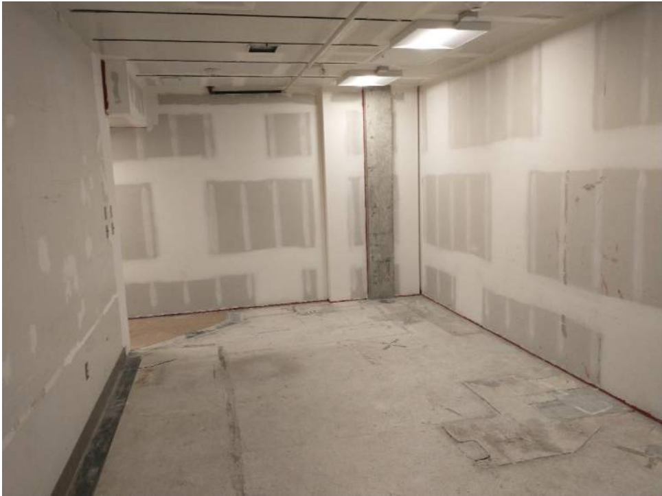
1 st Floor Vacant Space 1119 with exposed concrete column
