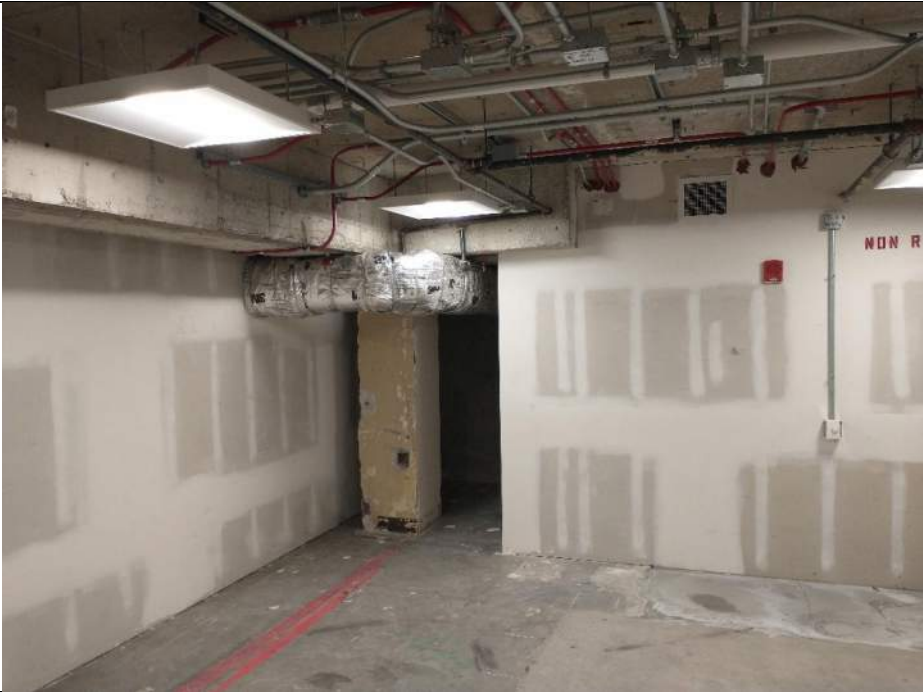
Ground Floor Shell Space 0102 with plaster finished column and exposed concrete beam and ceiling deck
