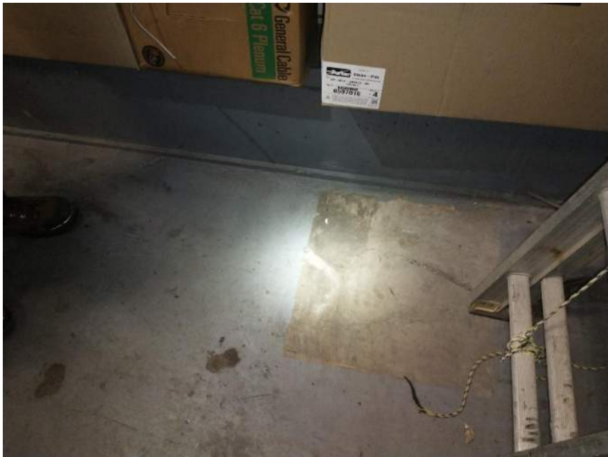
9 th Floor Mechanical Space 9100 showing no black floor mastic post wash
