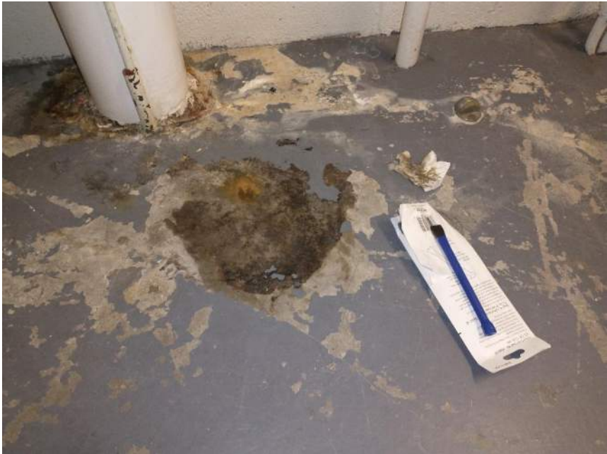
4 th Floor Mechanical Room 4144 post floor wash with black mastic visible at washed area
