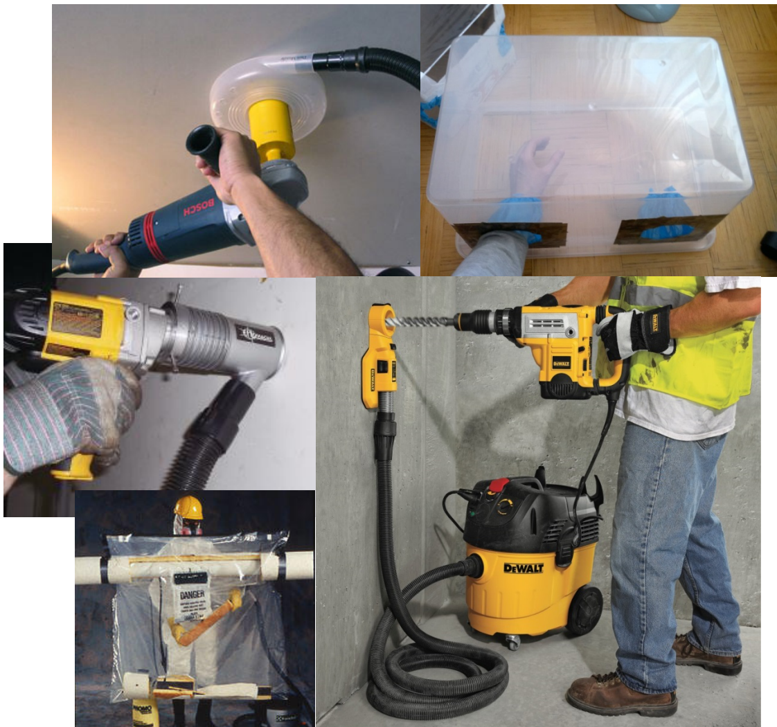
Examples of glove bag/box and HEPA shrouded systems
